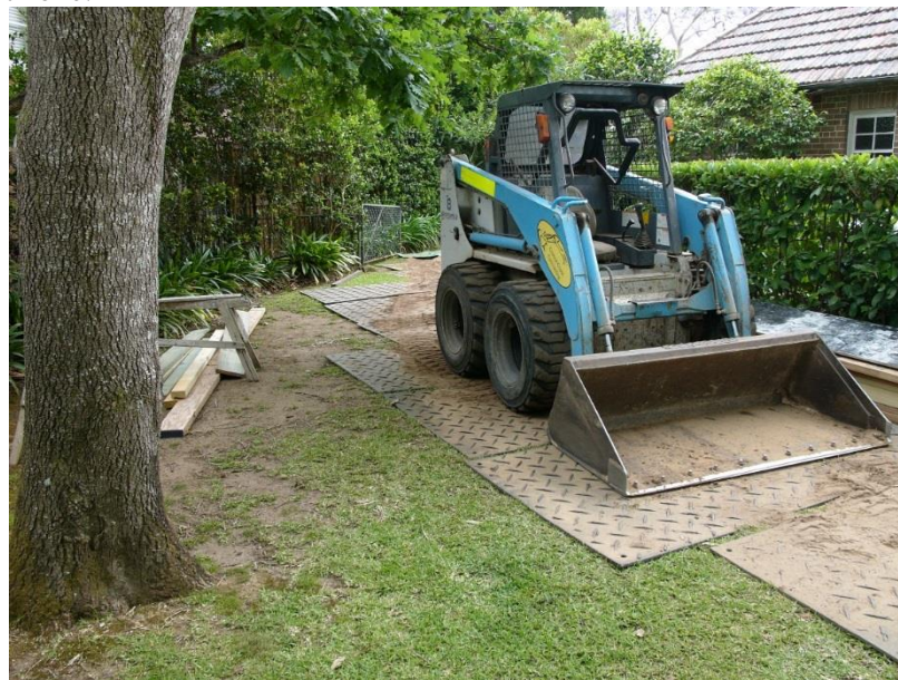
Figure 4 – Showing typical detail for truck mats.
